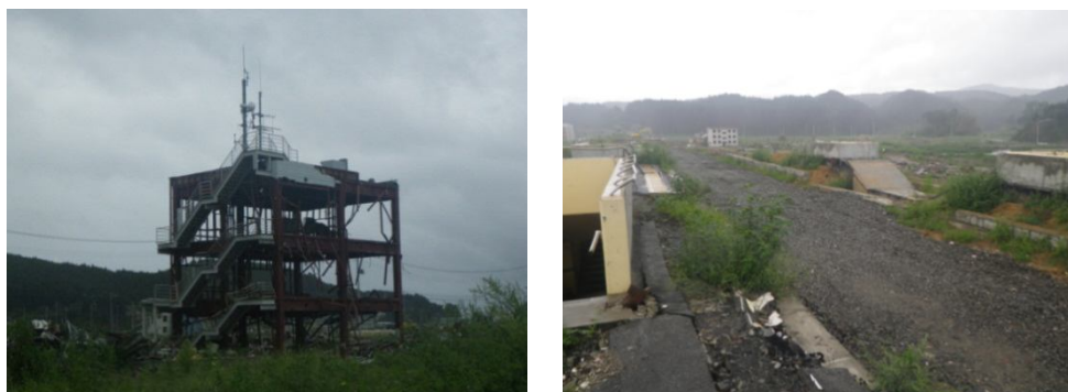
Fig. 8 Disaster prevention building (3/9/2011) and JR train station (3/9/2011)
